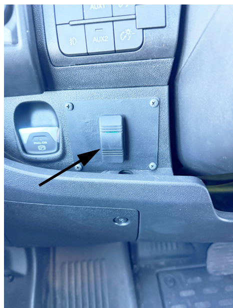
3. There is also a generator start/stop switch on the dash. -Typical View
