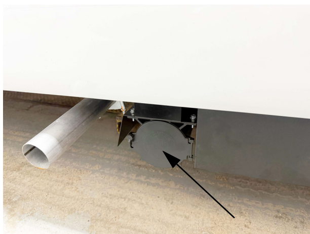
The sewer hose is stored on the driver's sidewall in this compartment. -Typical View
